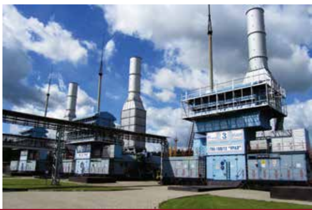
Gas Pumping Unit GPA-16 "Ural"
