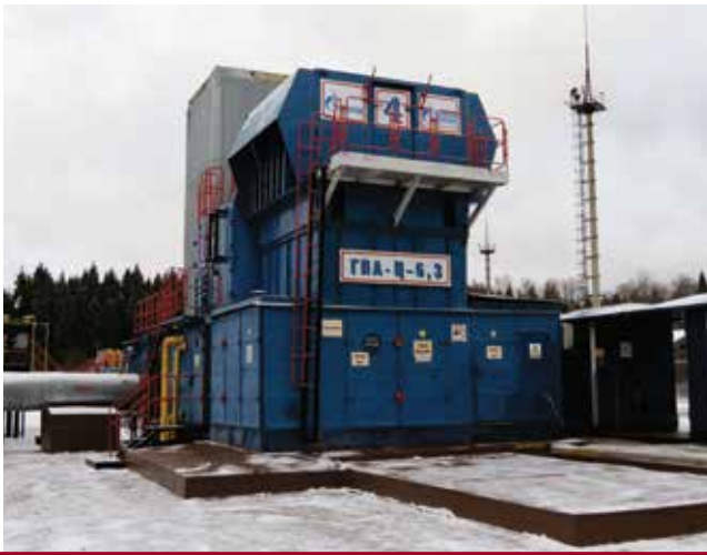
Gas Pumping Unit GPA-Ts-6,3
