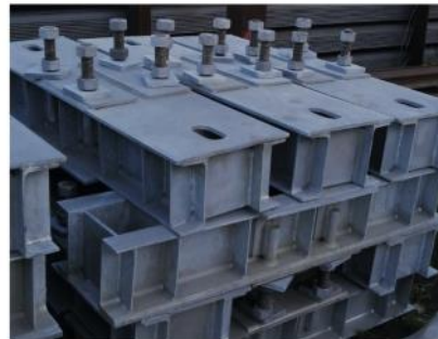
Pile foundations (grillage)
