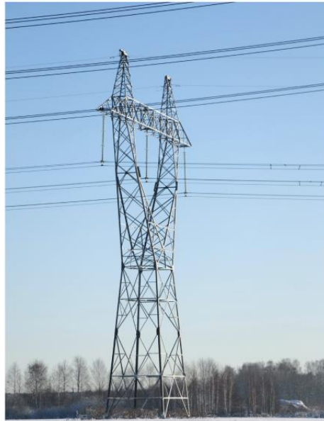
Metal structures of power transmission poles 35-750 kV, including supports of the new unification 220-500 kV
